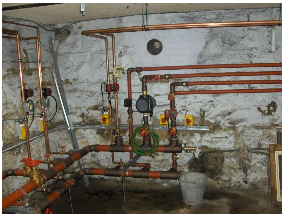
Zoning pipework, pumps and valves during installation
