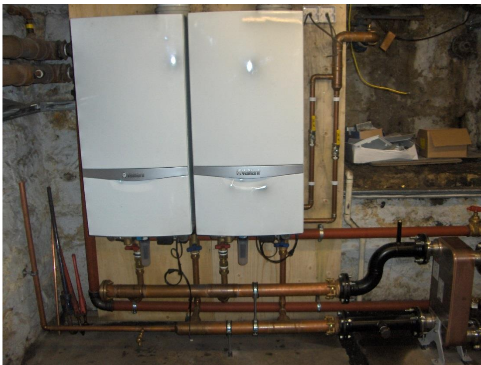
New Boilers and heat exchanger during installation
